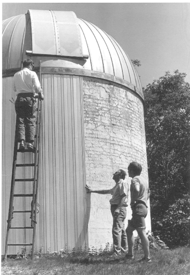
Left: Adding aluminum cladding to the observatory. Right, the 8-inch Spacek refractor.
